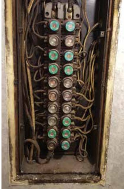
This old fuse box is loaded with obsolete wiring and it lacks adequate insulation.
